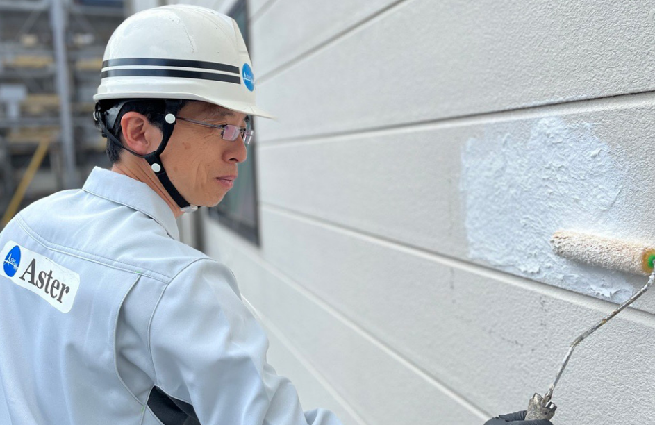
Left: SUZUKI Masaomi, CEO of Aster Co., Ltd., applies Aster Power Coating to a wall using a roller. ASTER Below: Aster Power Coating contains both glass fiber and acrylic silicone resin.
