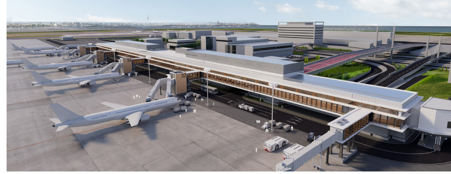
Digital rendering of the completed hybrid wood-steel structure used for the new north satellite facility extending from Haneda Airport Terminal 1. JAPAN AIRPORT TERMINAL CO., LTD.
