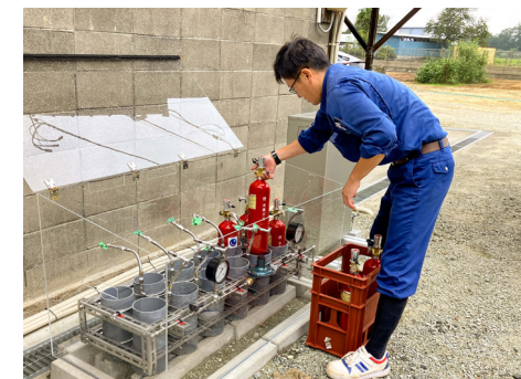
Left: Since September 2023, Namie has been implementing a pilot project delivering small cylinders—filled with hydrogen and weighing around 2 kg each—to ordinary residences and other locations. In this photo, a delivery driver is connecting the cylinder to a residential hydrogen fuel cell. Right: Although Namie's population decreased significantly—to approximately one-tenth of its former size, or 2,200 people—following the 2011 earthquake, it has already built two hydrogen stations and makes widespread use of FCVs. JUI
