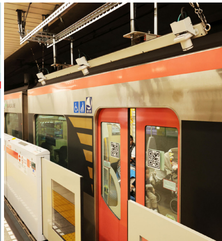
Left: A camera reads the data and movement of 2D codes attached to both train doors, signalling the opening and closing of the platform door. Right: The camera seen in the upper right of the photo reads information from 2D codes, such as the number of train cars and the position of the doors.
