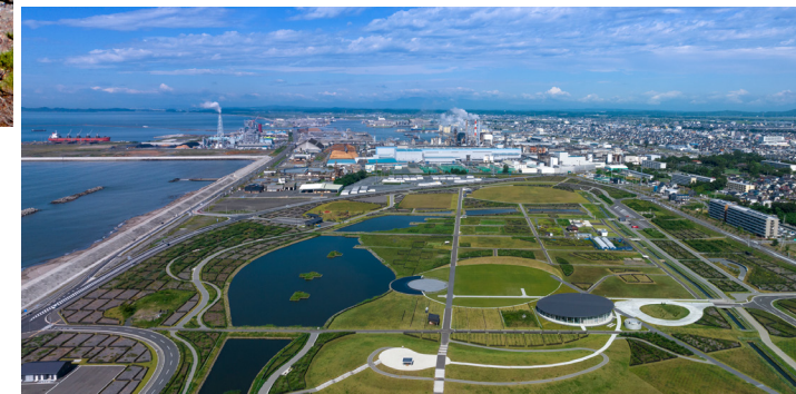
Left: Ishinomaki was among the cities most devastated by the tsunami of March 2011, with nearly 4,000 people either dead or missing. THE GREAT EAST JAPAN EARTHQUAKE ARCHIVE OF MIYAGI Above: Ishinomaki Minamihama Tsunami Memorial Park is located in a district that suffered extensive damage. The park opened in 2021 to commemorate the victims of the earthquake and tsunami, to pass on the memories and lessons, and to express the city's firm determination to rebuild, both at home and abroad. ARC IMAGE GALLERY/ AMANAIMAGES
