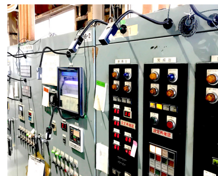
The IntegrAI system is ready to go after simply attaching a camera to an instrument.
