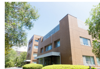
The facade of the Hiroshima University Research Institute for Nanodevices. Formerly named the Research Center for Integrated Systems, it was established in 1986.
