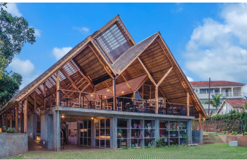
Tank Hill Park made use of local timber to create an open space. In 2020, the building was awarded the Good Design Gold Award (Minister of Economy, Trade and Industry Award) by the Japan Institute of Design Promotion as an outstanding example of Japanese design. TIMOTHY LATIM
