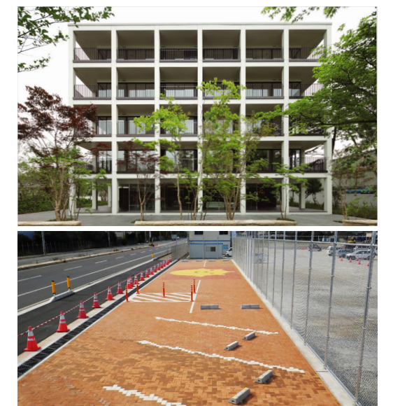
Top: In the field of architecture, the product is used in such places as the ceilings of apartment balconies (photo). Since its dense surface prevents water intrusion, concrete skeletal structures can be effectively protected, even in areas exposed to the elements. KAJIMA CORPORATION Bottom: The CO 2 -SUICOM products are currently made at precast concrete plants with special equipment. Among the concrete’s main applications are paving blocks in parking lots (photo) and road demarcation blocks. KAJIMA CORPORATION
