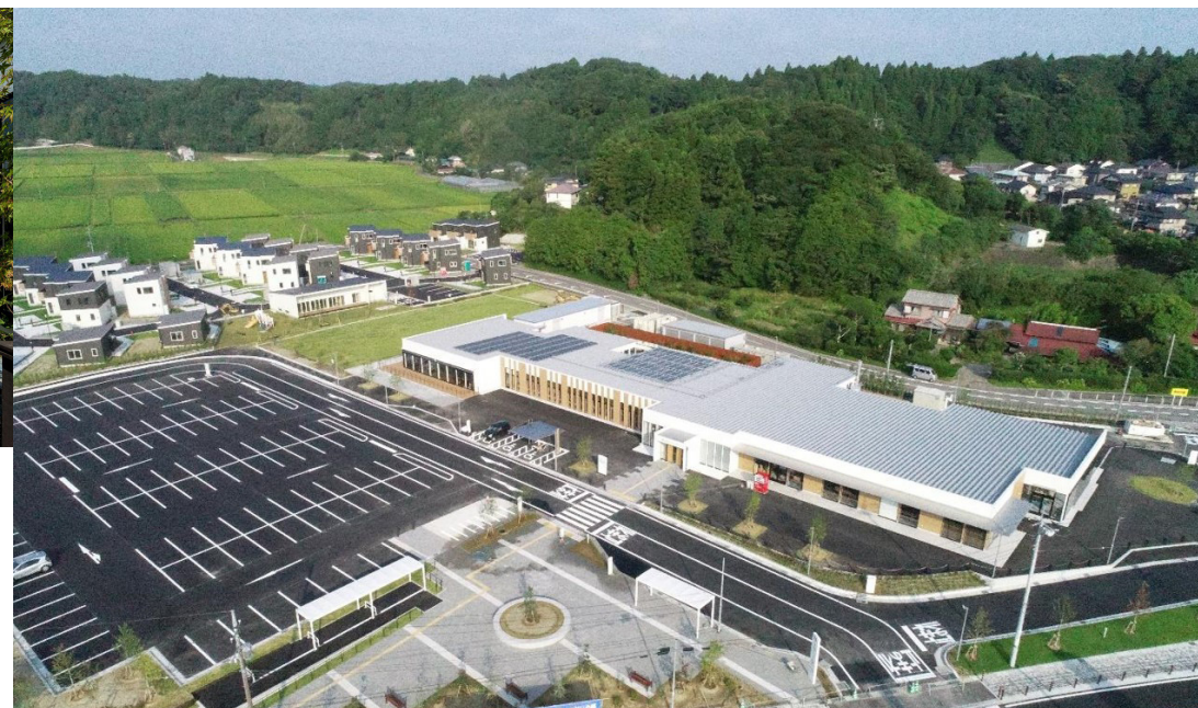
Top: The region was plunged into darkness by the 2019 typhoon, but the roadside station was able to turn on its lights and provided relief to neighboring residents. Left: Mutsuzawa Smart Wellness Town established a cogeneration system using locally produced natural gas and a microgrid of locally operated power lines. The roadside station has also installed solar power generators.
